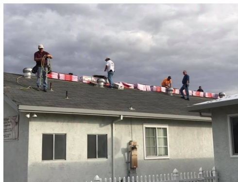
Reroof sanctuary and parsonage in Woodbridge
